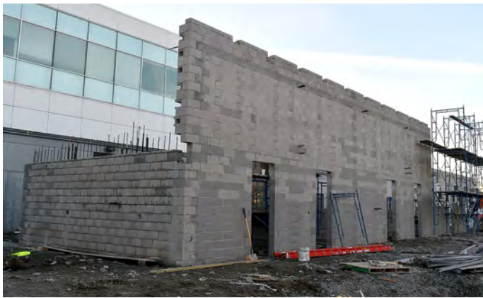
Equine expansion construction in November 2025 Photos: Dave Gieseke
